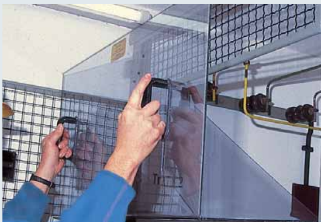
Inserting a transparent insulating protective shutter of type A2
