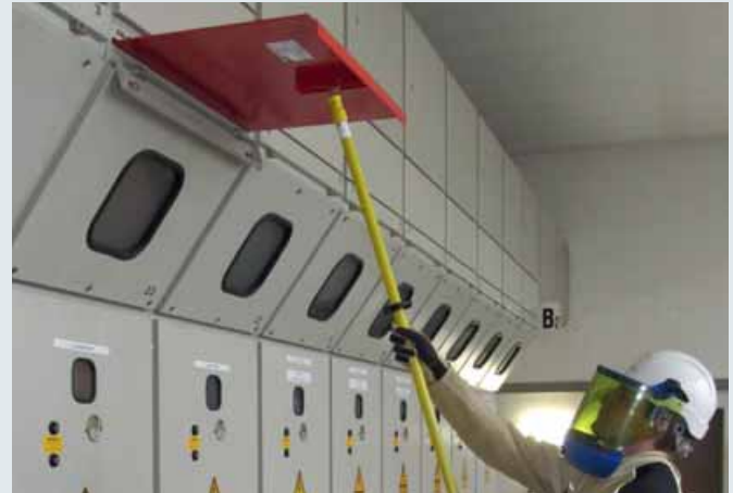
Inserting an insulating protective shutter of type A3 by means of an operating stick
