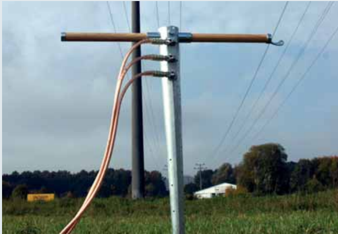
Earthing busbar and earthing cables mounted on a tubular earth electrode
