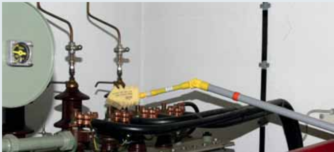
TFRS MS combined cleaning kit used for dry and damp cleaning of a transformer under live conditions
