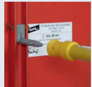
Inserting an insulating protective shutter of type A3 by means of an operating stick
