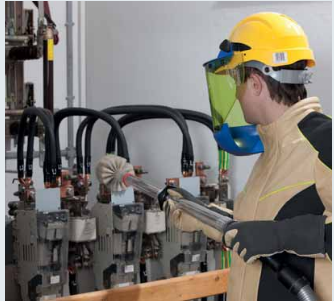
Live cleaning of a transformer using the TRS MS dry cleaning kit
