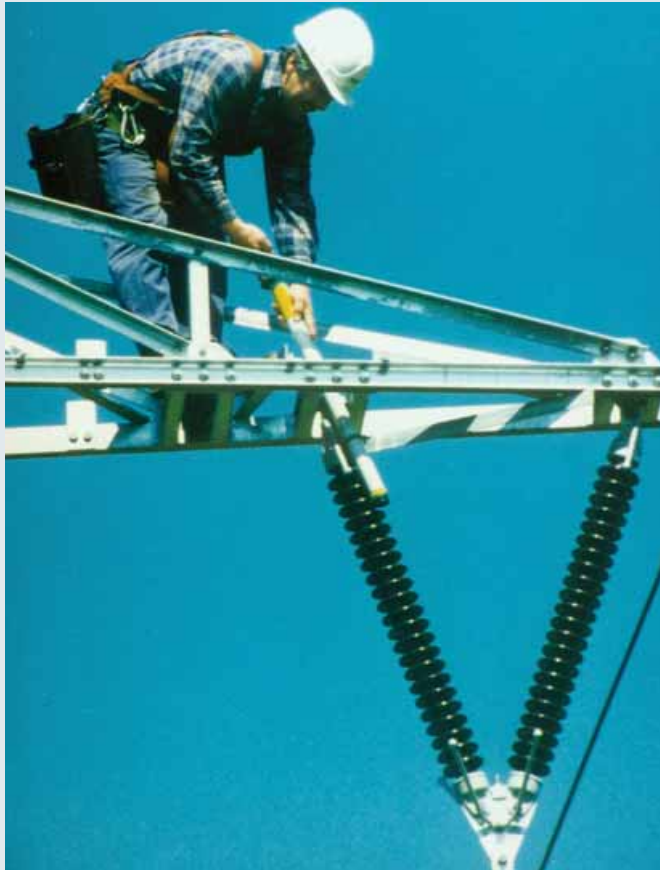
Non-contact voltage detector used on a 110 kV overhead line
