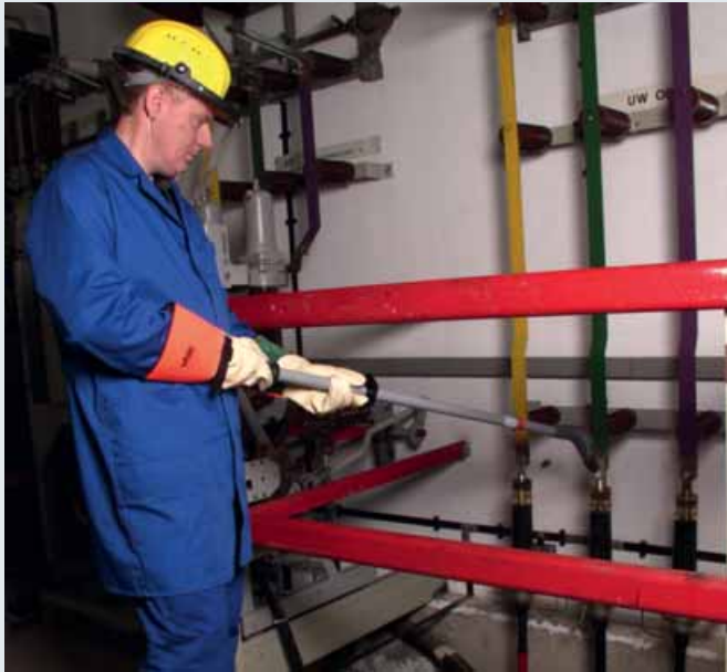
Loosening a screw plug using the MS insulated screw driver
