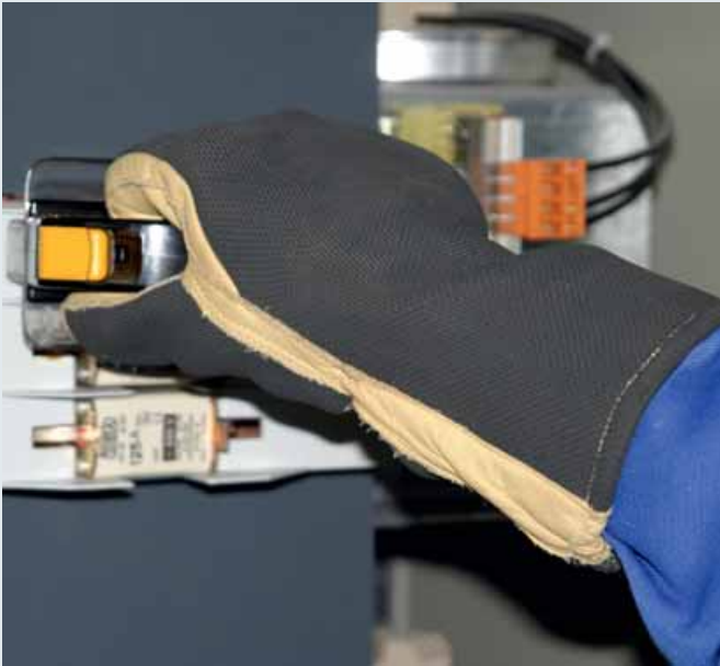
Actuation of an NH fuse puller using protective gloves
