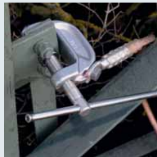
Earth milling clamp attached to a varnished steel mast
