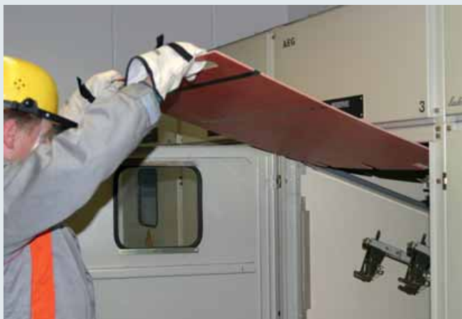
Inserting an insulating protective shutter of type A1
